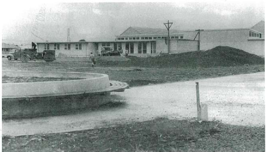
School nearing completion
